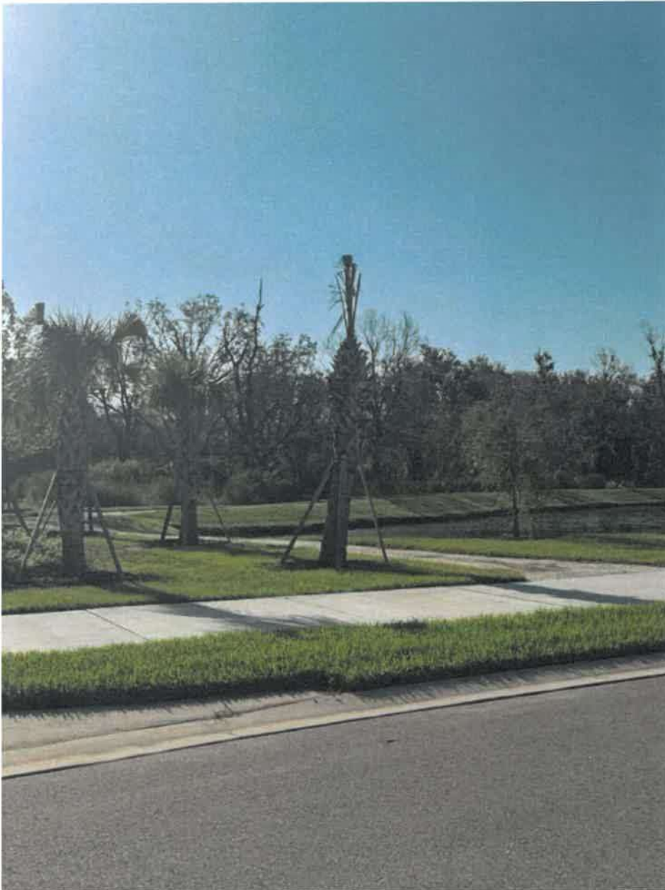
Spruce River way lift station
